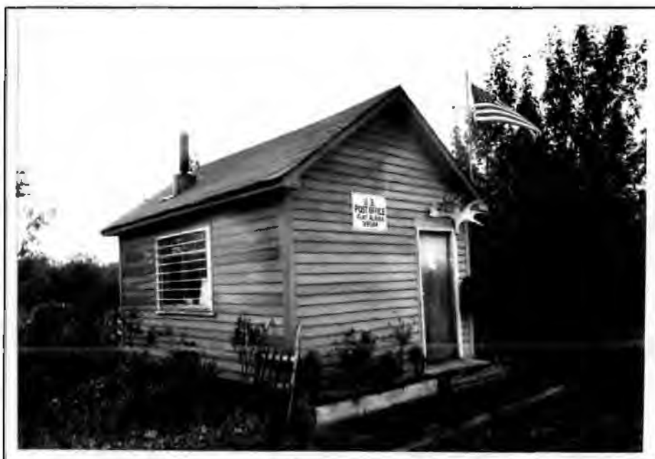
Figure 91. The Post Office Building, 1993. The view is looking northwest.
